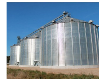
钢板仓 Steel Silo
